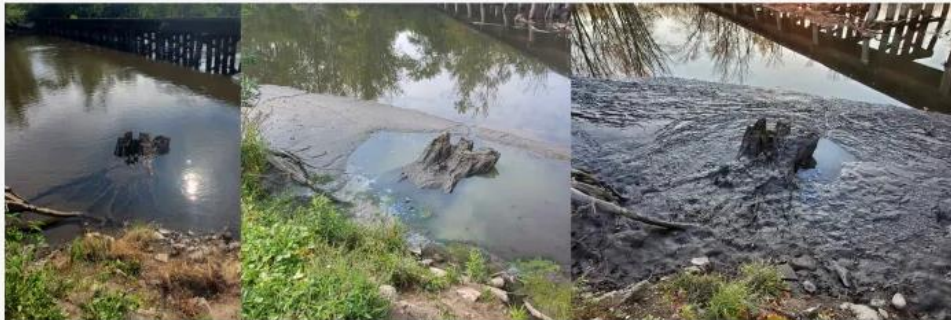
Progressive sludge build-up on one bank. Each photo was taken two months apart from the other. Photo by: Ryan Baker
